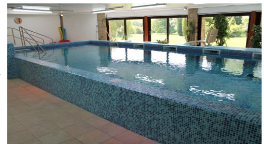
An example of a semi-raised freeboard pool
